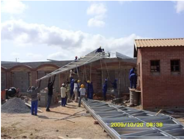
Hoisting the trusses
