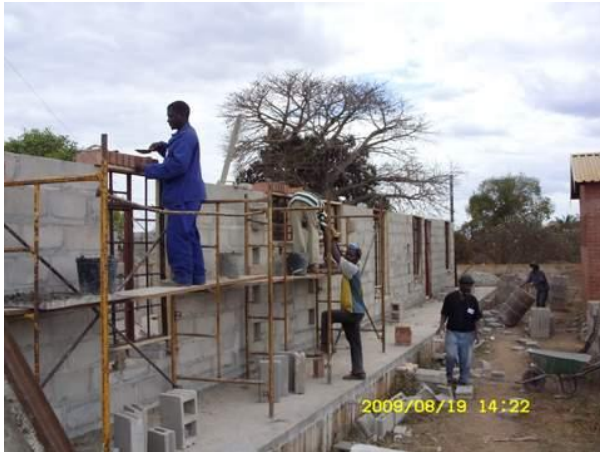
Erecting the rear wall of the building
